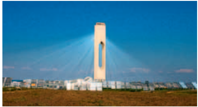
The PS10 test facility in Seville, in southern Spain with an electrical capacity of 11 megawatts, demonstrates the possibilities of solar thermal tower power.
